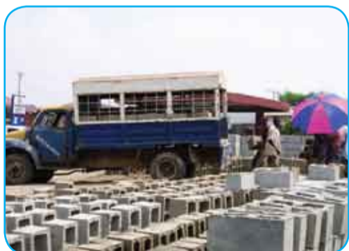
This bricklaying business in Ibadan, Oyo State is run by one of BIMFB's SMME customers.
