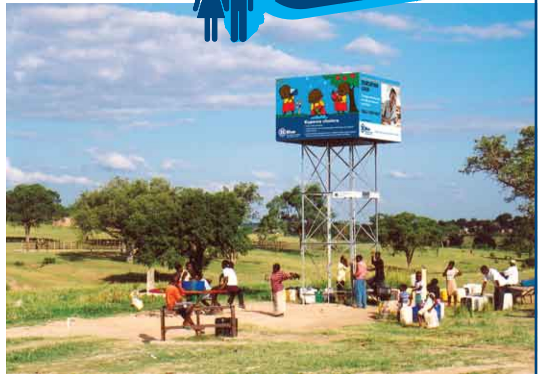
The PlayPump water system, which provides easy access to clean drinking water, all while bringing joy to children; displaying Blue's signage.
